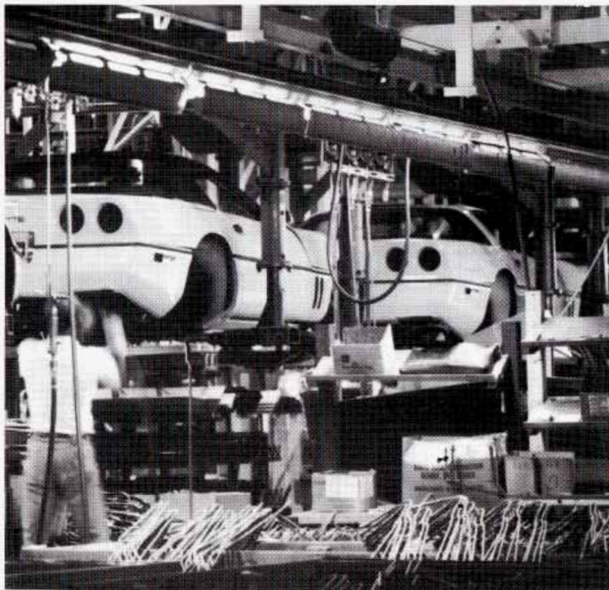
The Corvette Assembly Plant in Bowling Green, Kentucky, is one of the most sophisticated and computerized automobile assembly facilities in the world. To build your 1994 Corvette, over 1,200 employees teamed up with the 70 high-tech robots that assist in a variety of processes, from welding to painting.
